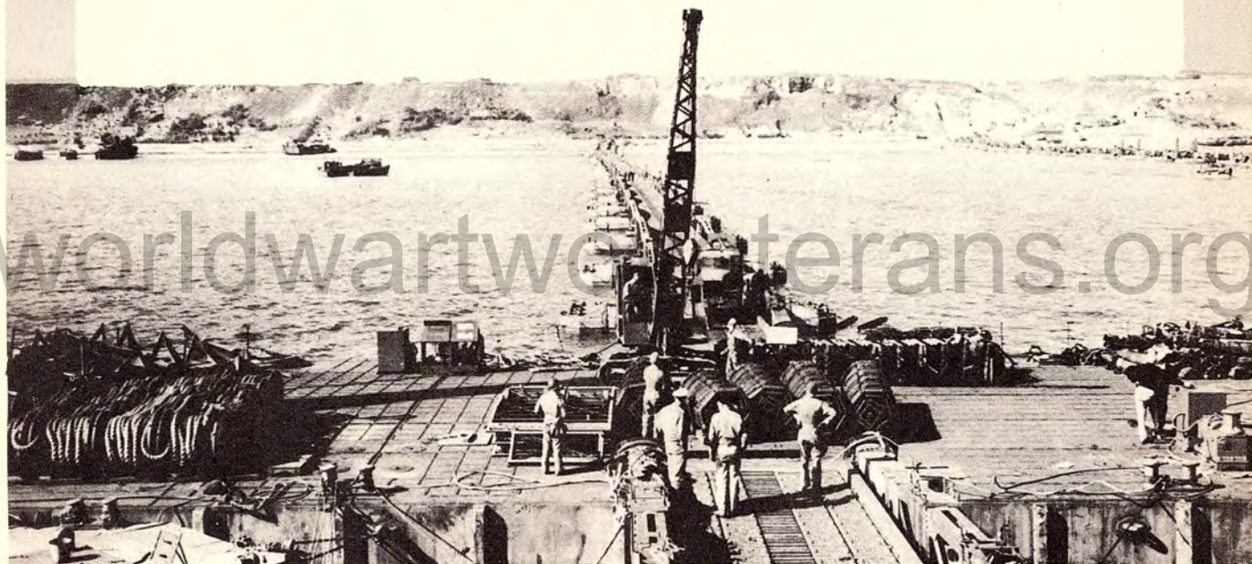
"MULBERRY"--THE SECRET FLOATING HARBOR, NORMANDY LANDINGS Large concrete or steel pontoons were installed at regular intervals transverse to the pontoon bridgeway to strengthen it and to serve as mooring places for vessels. Omaha beach can be seen in the background.
